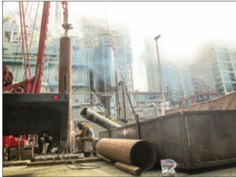
A driller welding casing on the Seattle project
